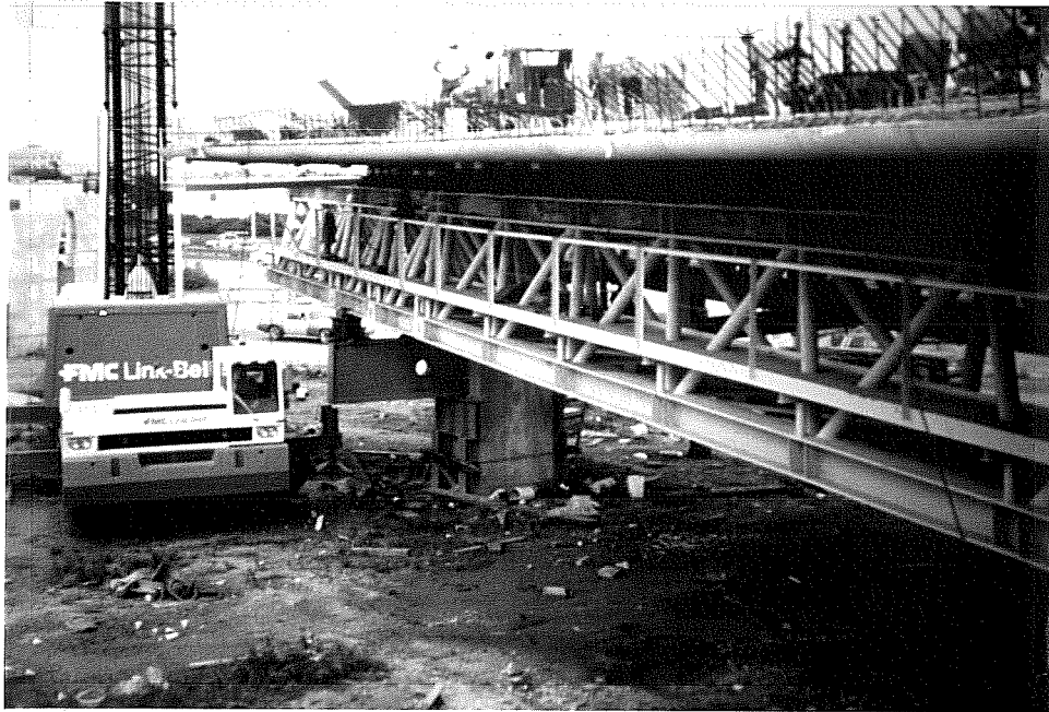
Figure 1.24 Austin Bridge Company's erection truss.
