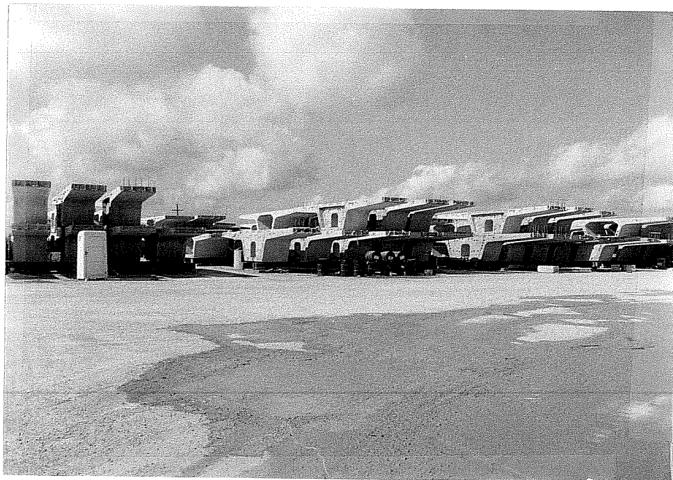
Figure 1.23 Storage area in casting yard.
