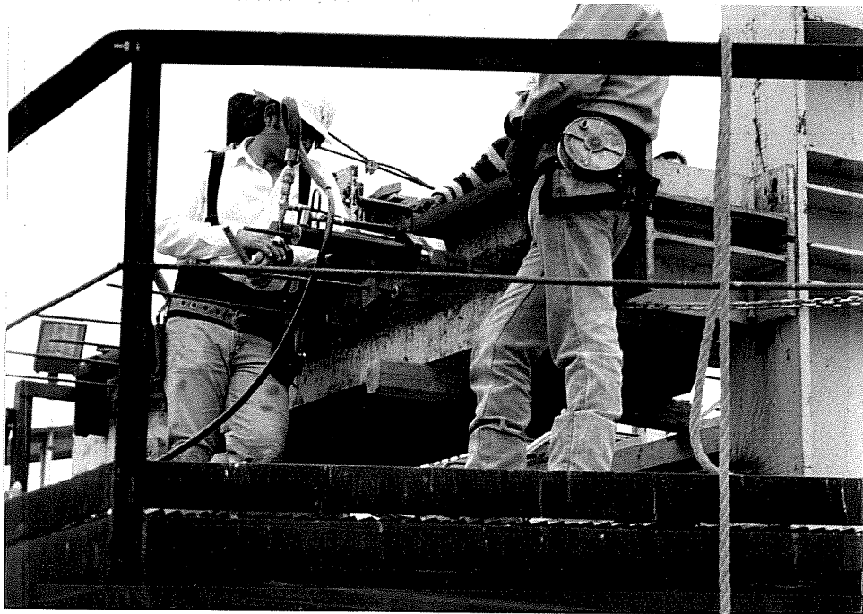
Figure 1.20 Prestressing of transverse tendons in casting bed.
