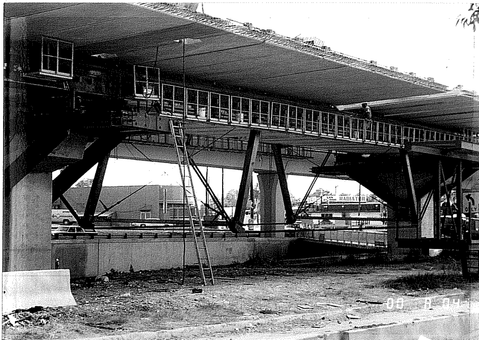
Figure 1.25 H. P. Zachry Construction's erection truss.
